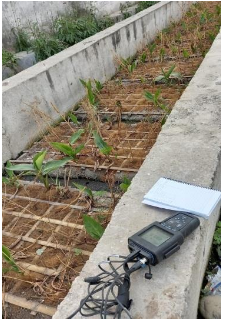
Fig. 1b Floating constructed wetlands for in-situ treatment of domestic wastewater in urban drain.
