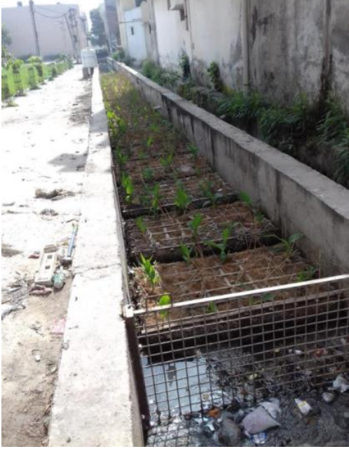
Fig. 1b Floating constructed wetlands for in-situ treatment of domestic wastewater in urban drain.
